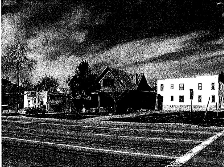
6th and 6th Office Building (Original Conditions)
